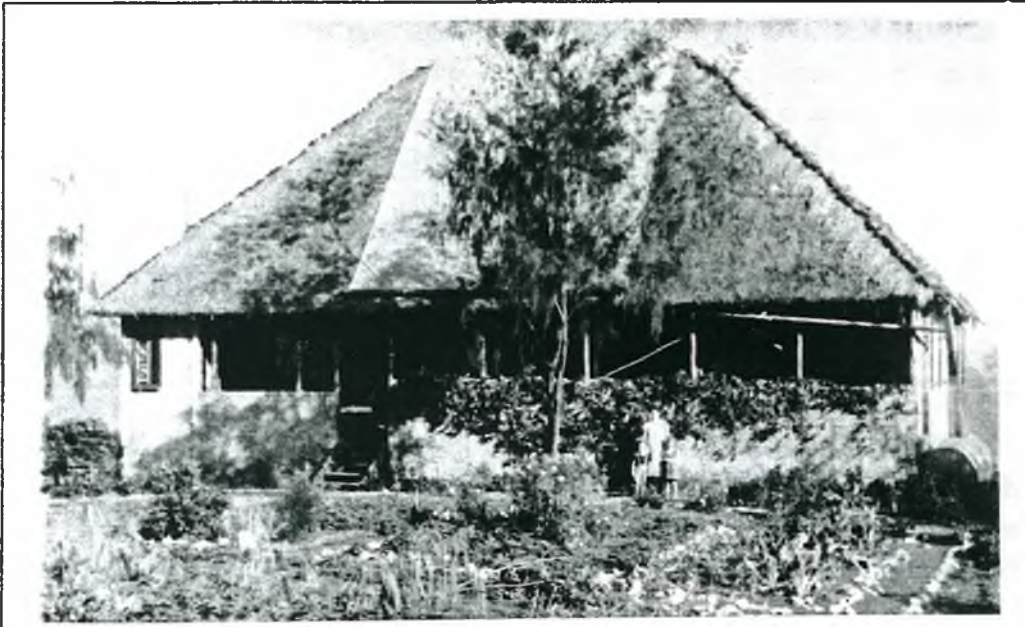
The Stafford house at Kumul contained woven bamboo walls, a kunai grass roof and a hand planed floor. March 1952
